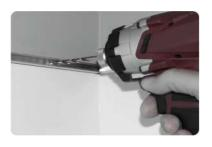
Hold U-channel in required position and drill pilot holes through the channel and into your liner/tiles. A small amount of silicone can be applied to holes and along the length of the U-channel to improve water tightness prior to screwing bracket on.
