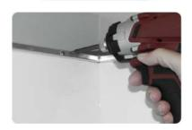
Using screws provided, attach U-channels to the shower wall.
